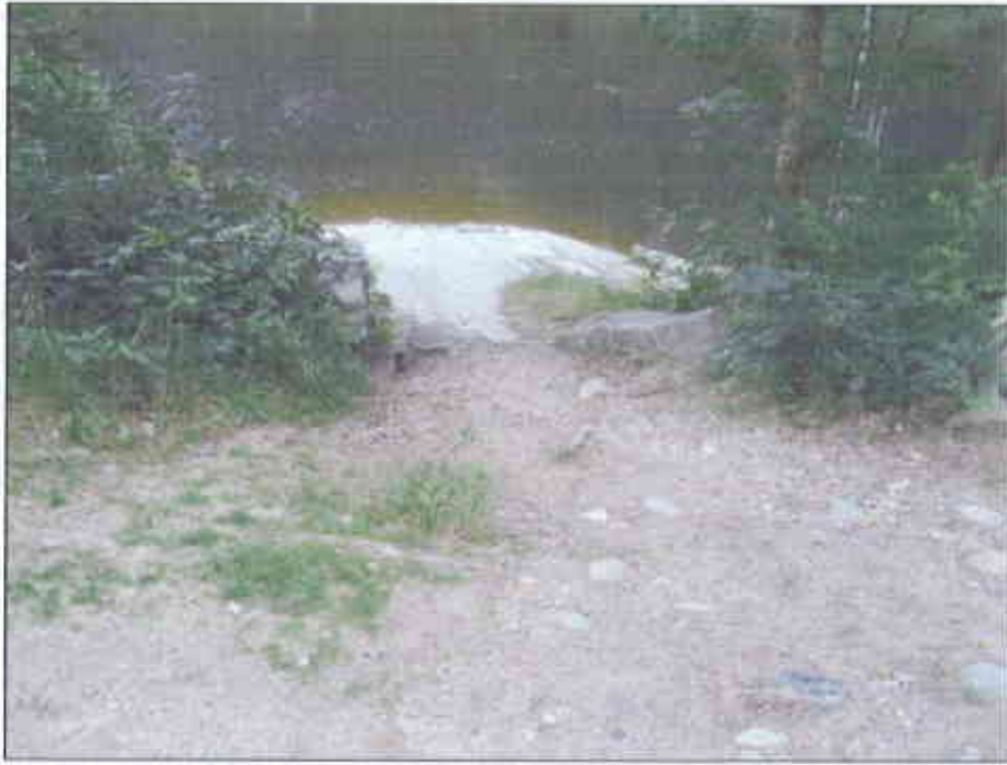
Route 181 East Shoulder with Gully Erosion
