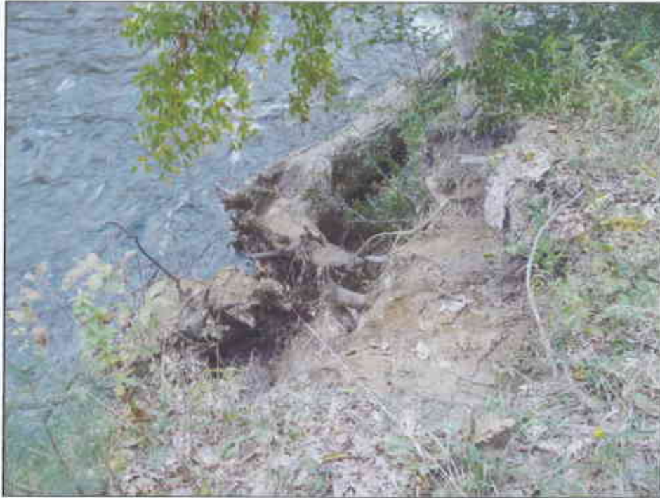
Bank Instability observed along the right (west) bank of the Farmington River
