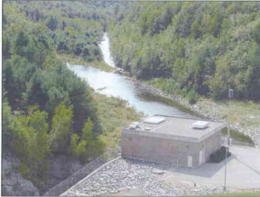
Segment 1A Hogback Dam tailrace with bifurcated channel
