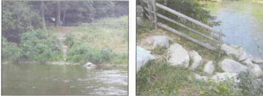
Log Revetments and Natural Stone Stairways constructed along the river.
