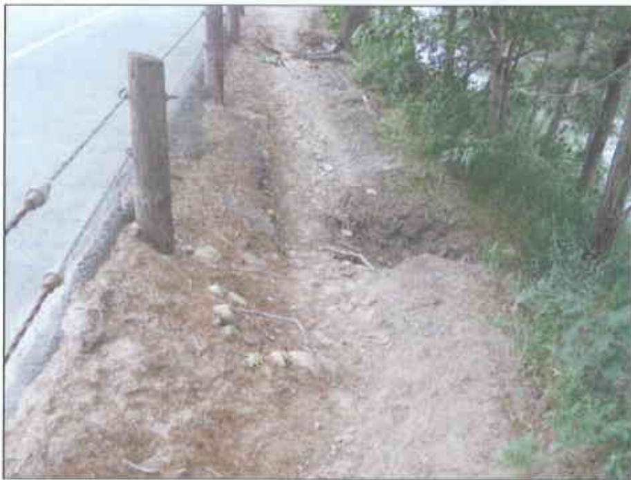
Route 181 East Shoulder with Gully Erosion
