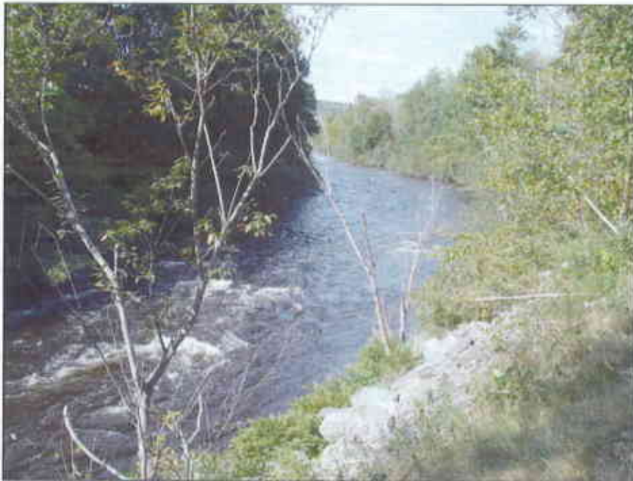
Vegetation and riprap armament located within Segment 1A along the left (east) bank of the Upper West Branch
