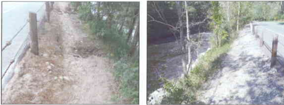
Gullies resulting from sheet flow runoff along nearby roads.
