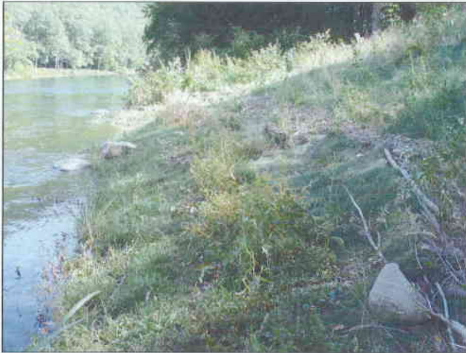
River banks well vegetated and stable at the Tennessee gas pipeline crossing
