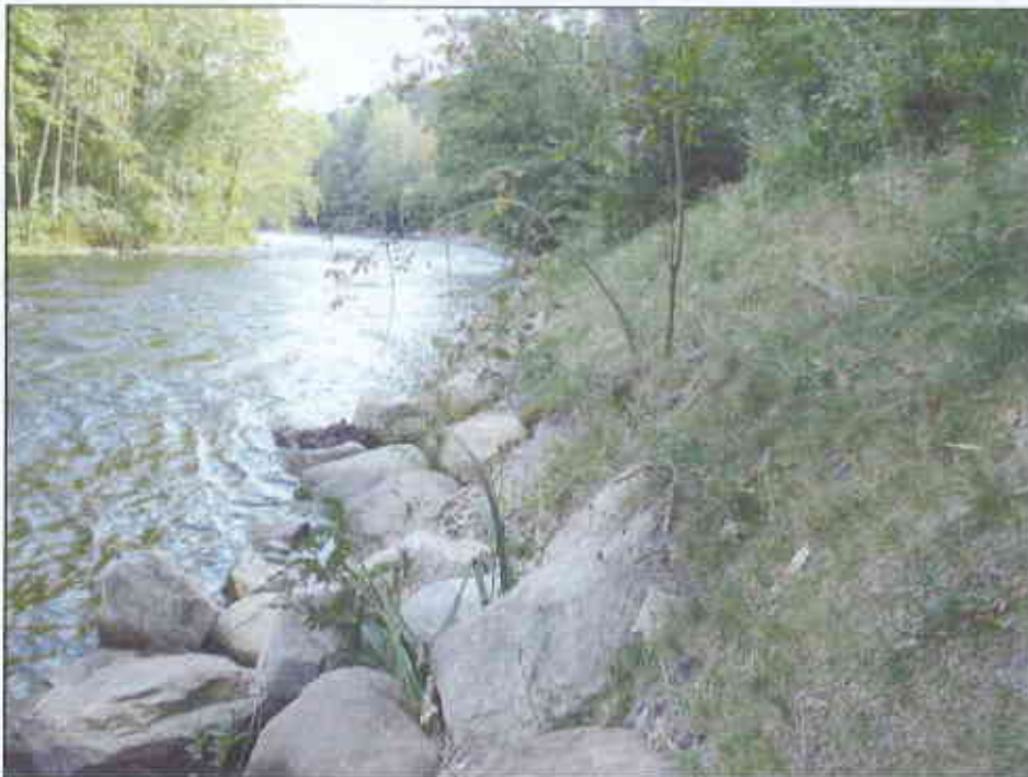
Bank stabilization project located within Segment 1B illustrating rock armament at rivers edge with well vegetated, stable banks.
